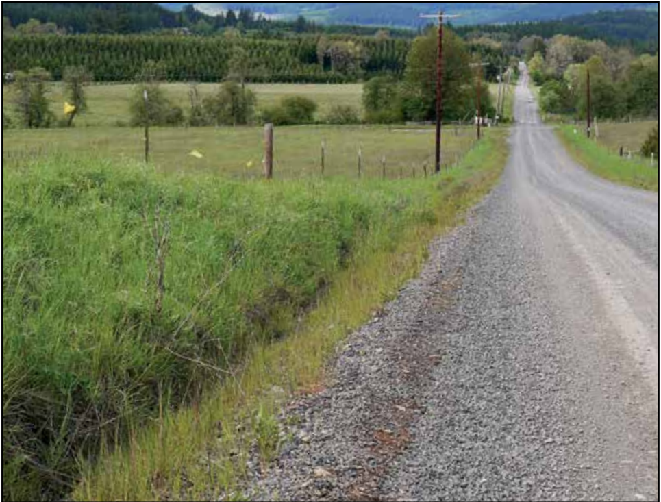
Maintaining a good surface on a gravel road involves grading, which smooths the road by scraping it. In the process, plants growing on the road side of the ditch can be buried, along with any butterfly eggs or caterpillars. Photograph by Bruce Newhouse.
